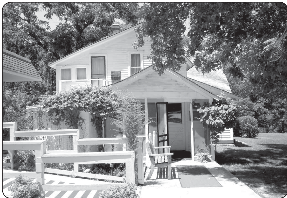
The back porch and entry to the kitchen at the farm house on the Wilder Home and Museum in Mansfield, MO. Museum steps are on the left. CONNIE PETERSEN PHOTO
